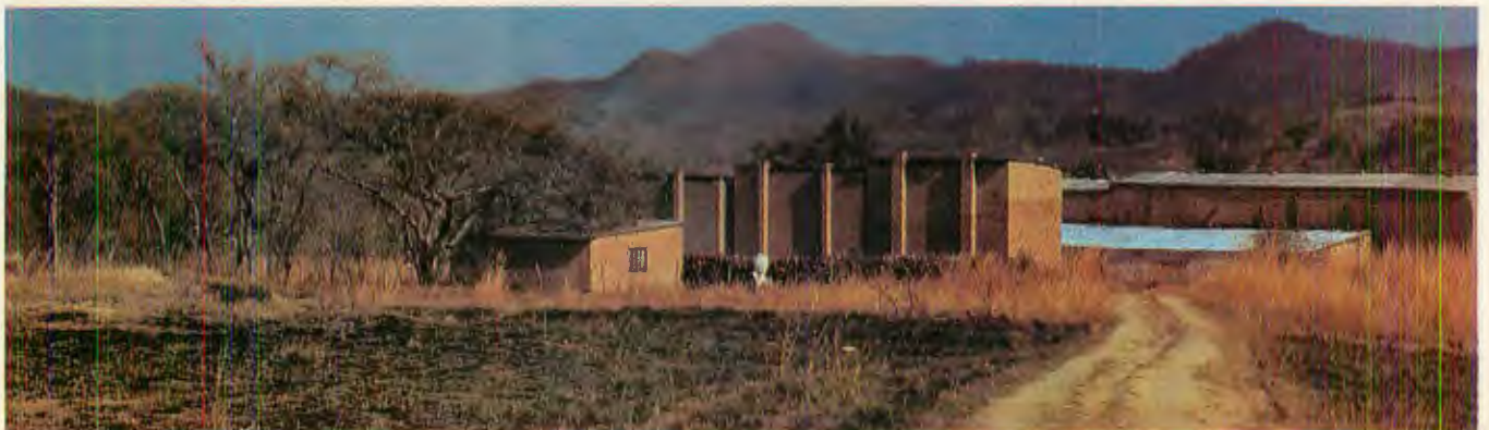
Tobacco barn and sheds on a farm near the Weya Tribal Trust Lands, showing the results of a brush fire assumed started by poachers.
